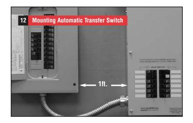
12. Locate automatic transfer switch with built-in emergency load center within one foot of main distribution panel. The automatic transfer switch can be located to the left or right of main distribution panel. Hold transfer switch against the mounting surface. Level the transfer switch and mark the mounting holes. Drill the appropriate size pilot holes. Mount the automatic transfer switch to mounting surface with appropriate fasteners.
